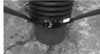
3. Take any excess strapping and loop the strapping through the ratchet piece and then close the ratchet.
