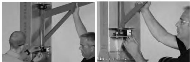
7. Line up Bearing holes with Support Bracket holes and secure Boom Bearings to Stack Support Brackets using 3/4" hardware supplied.
